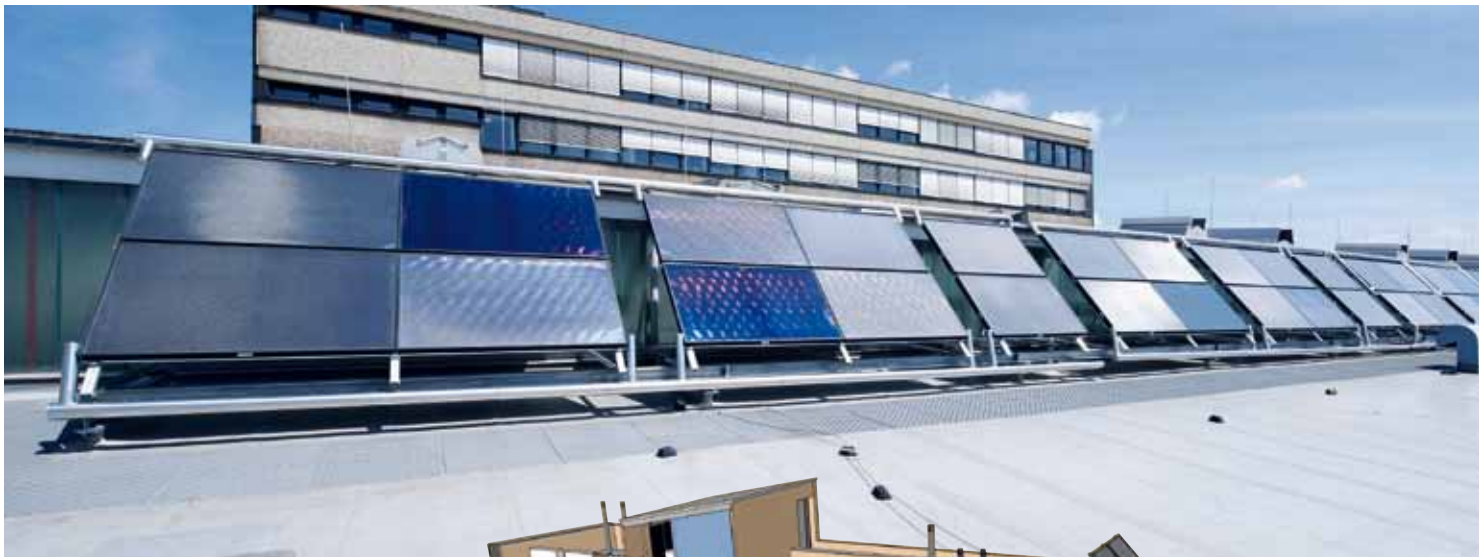
Vaillant flat-plate solar collectors provide the hot water supply for a pipe cleaning station at our Remscheid plant.
