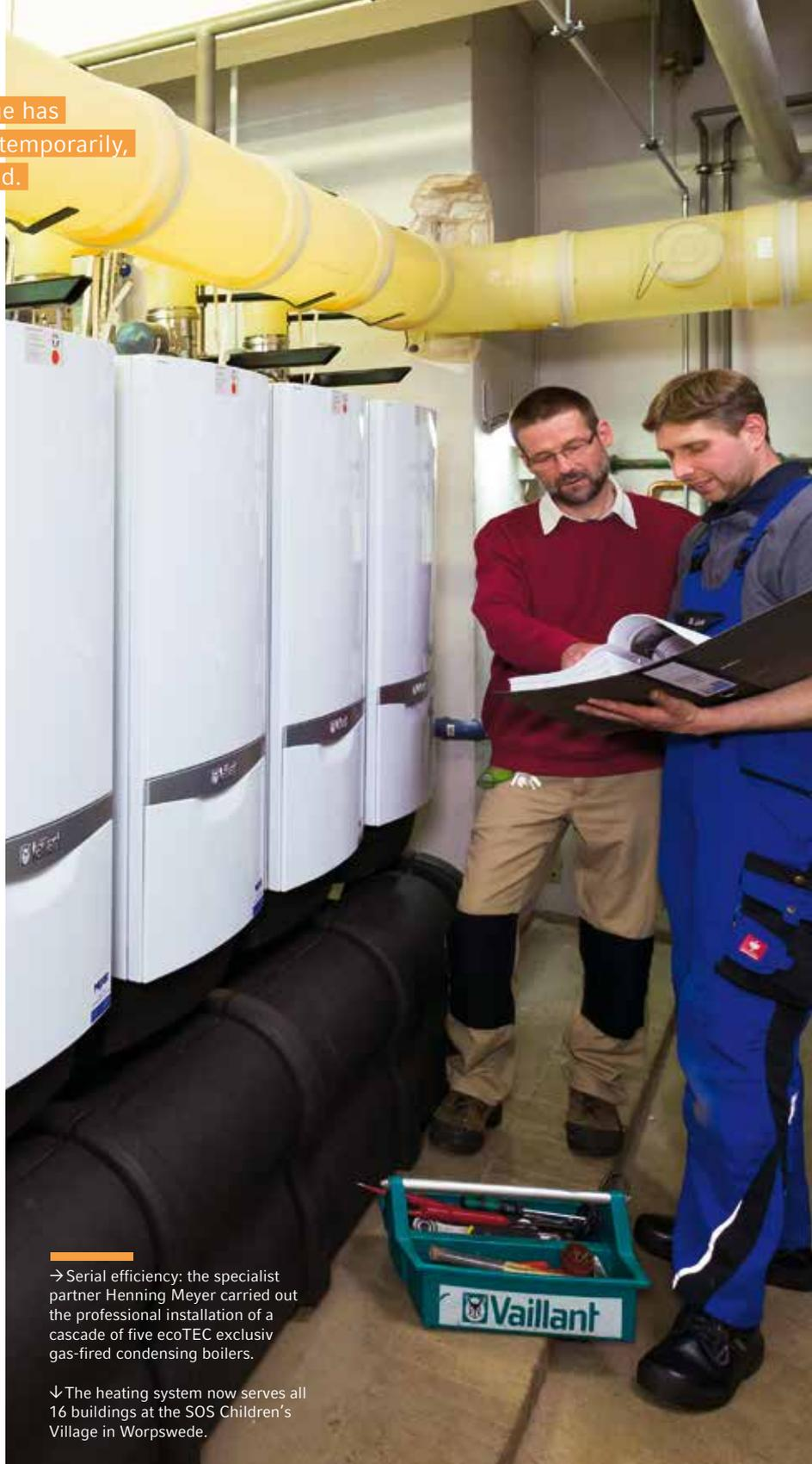
→ Serial efficiency: the specialist partner Henning Meyer carried out the professional installation of a cascade of five ecoTEC exclusiv gas-fired condensing boilers.
